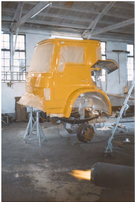
New front springs; and reconditioned and strengthened front axle installed.
