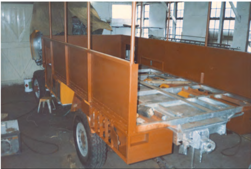
All lockers and tanks installed. Primer applied.
